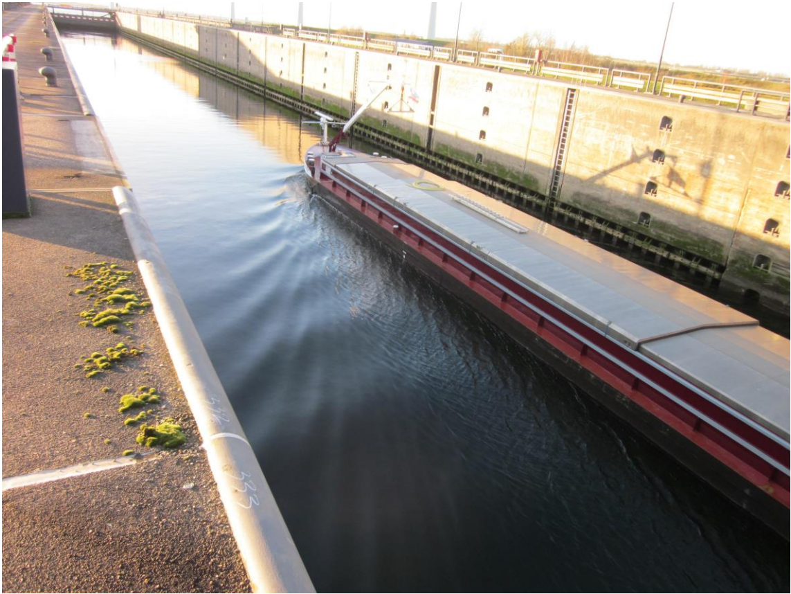
Figure B.7: Incoming vessel at the Krammer locks.
