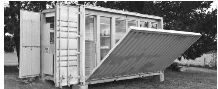
Case Study Port-A-Bach, dynamic openings being used to close up the house for transport.
