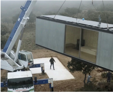
[Figure 74 & 75] TINI LIVING M, Being places on site in a Crane
