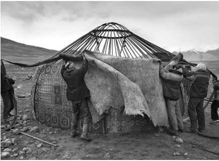
[Figure 2] Construction of a Yurt.
