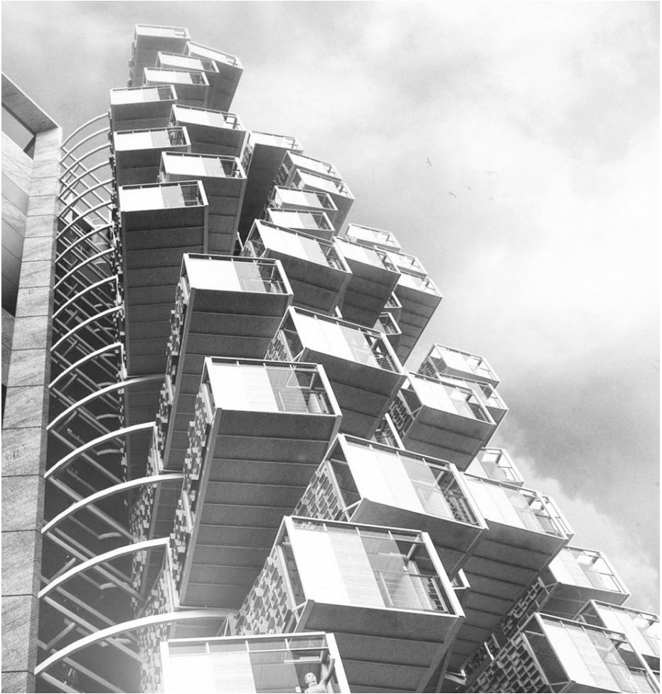
[Figure 43] Portable housing Project
