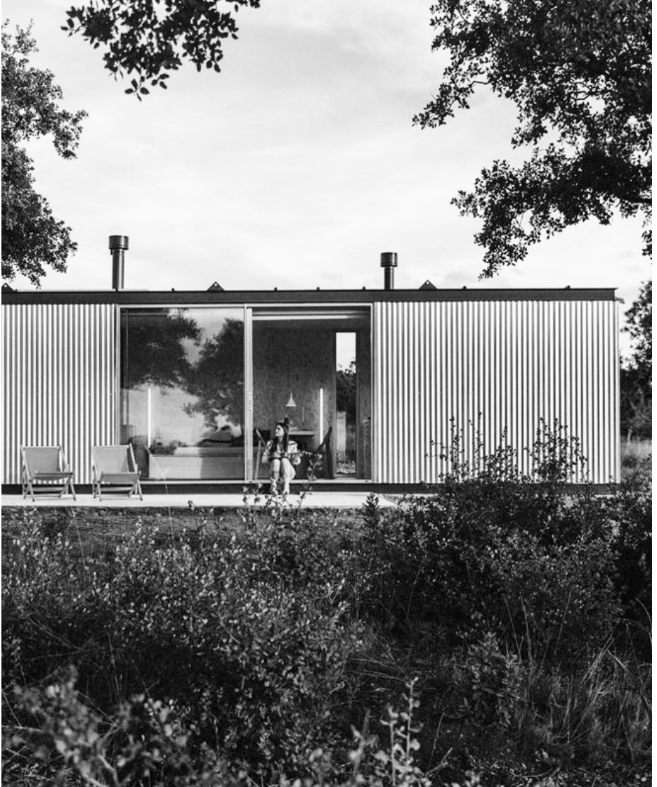
[Figure 76] TINI LIVING M, on Site
