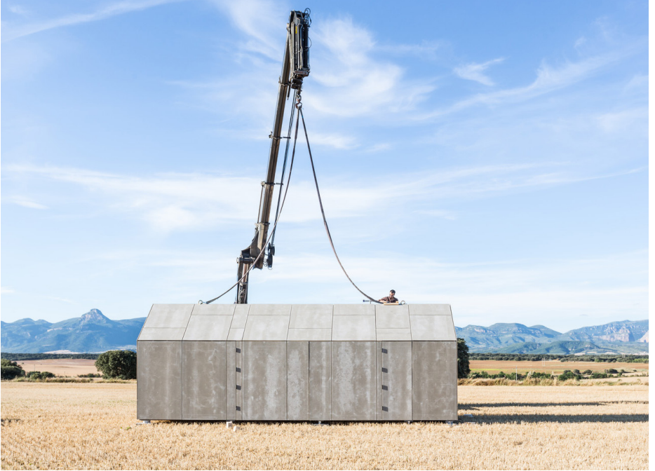
[Figure 69 & 70] ÁPH80, being transported and placed on site
