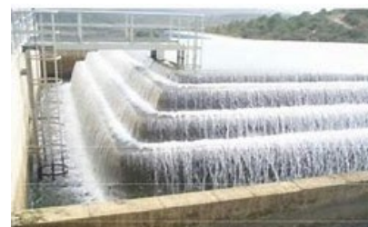
Figure 7: Cascade aerator (Ketav Consultant, n.d.)
