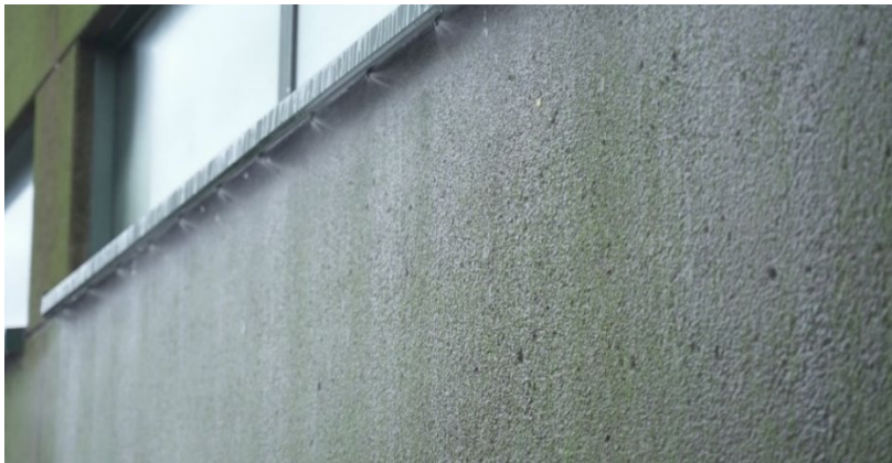
Figure 5: Respyre's current irrigation system. Spray nozzles can be seen underneath the window. On the wall below, wet and dry spots can be seen, indicating a non-uniform water distribution.
