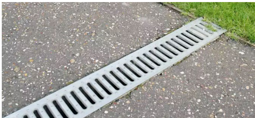
Figure 11: Channel drain (Wallender, 2022)
