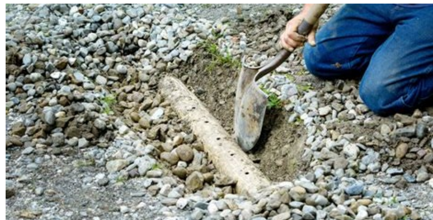
Figure 12: French drain (Ahrens, 2022)
