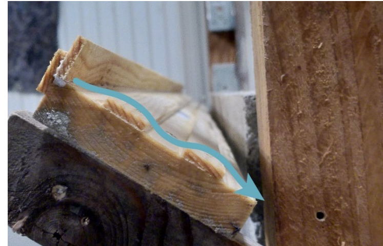
Figure 37: Gutter plank with ribbed surface.
