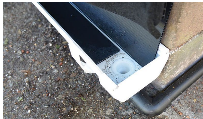
Figure 10: Gutter which collects water at the bottom of the wall. (Florafelt Living Wall Systems, n.d.)
