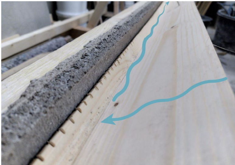
Figure 36: Gutter plank with ribbed edge.
