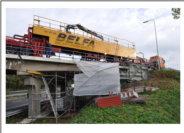
Figure 1. The German BELFA load testing vehicle on the Vlijmen-Oost viaduct in the Netherlands. Reprinted with permission from (1).
