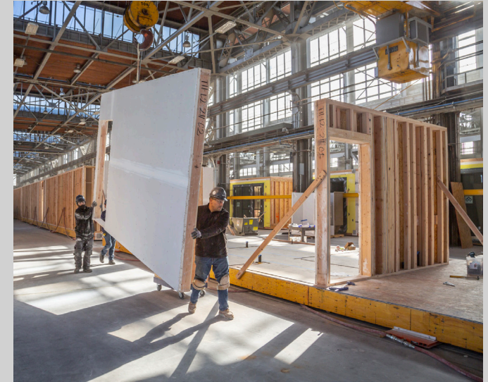
Developing construction technologies
