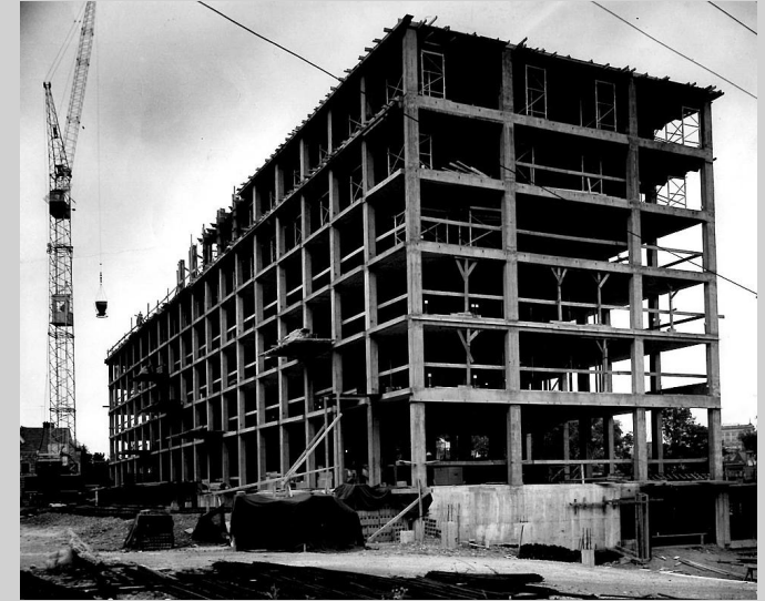
Developing construction technologies
