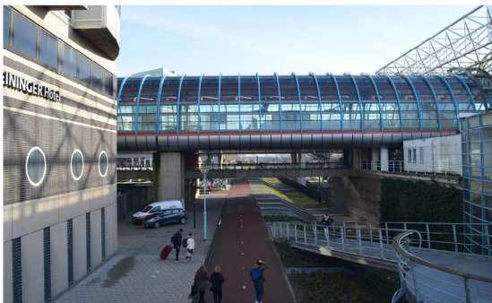
Level 1 to level 0 view, underpass Sloterdijk. (Owen source)
