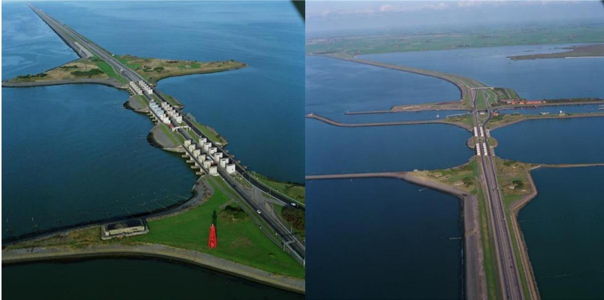
Figure 3: Sluice complexes at Den Oever (left) and Kornwerderzand (right)
