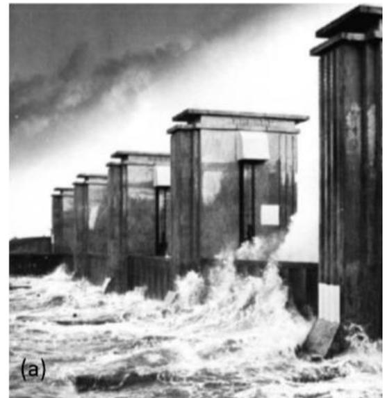
Figure 4: Wave impacts on the defence beams of the old sluice gates of the Afsluitdijk (Thijsse (1972))
