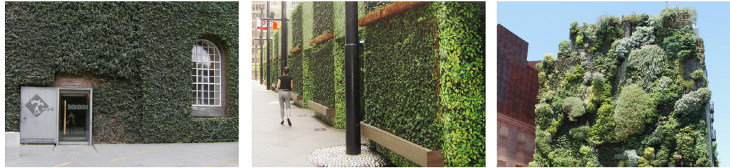
FIG. 2 From left to right: direct green façades, indirect green façades, living wall system (Manso & Castro-Gomes, 2015)
