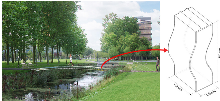
Figure 1 Aspect of the Glass Masonry Bridge and the brick shape
