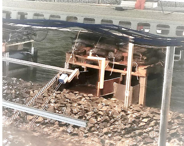
Figure 3. General layout at the entrance of an overtopping reservoir (run-up wave gauge, acoustic wave gauge to identify overtopping events, graduated staff).
