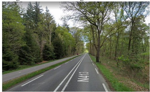
overgrown roadsides verges
