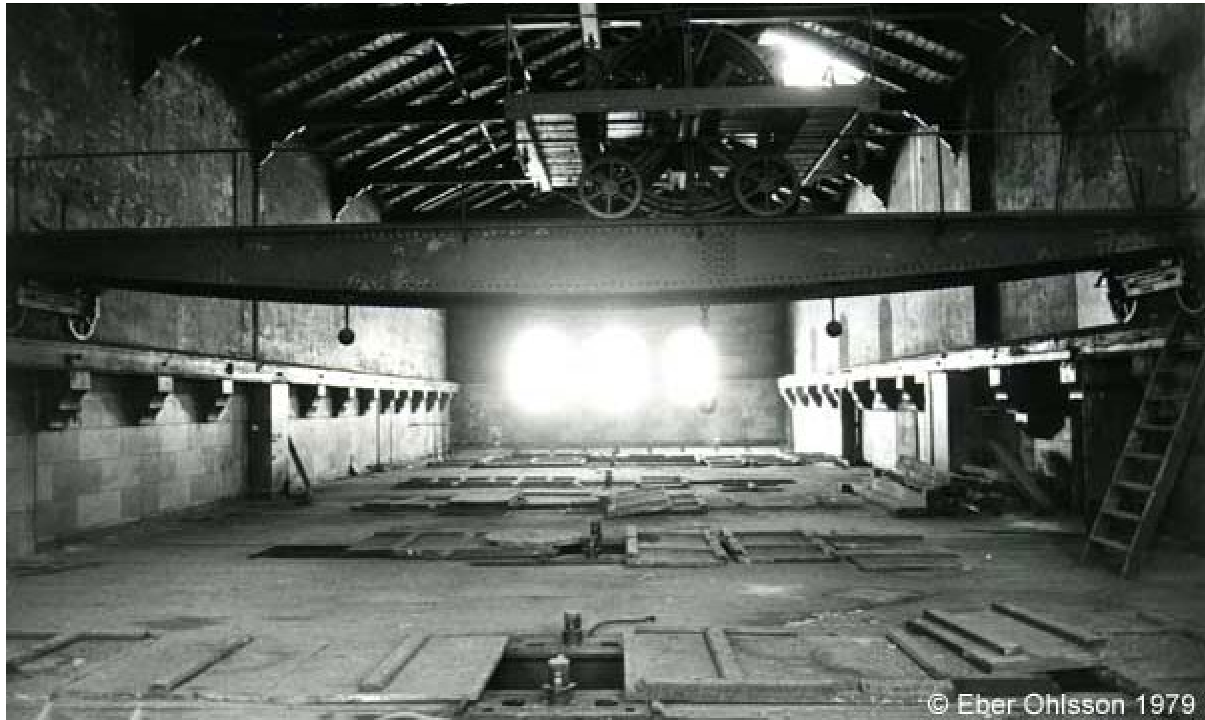
Pumphouse in the Site Copenhagen's Waterworks Outdated
