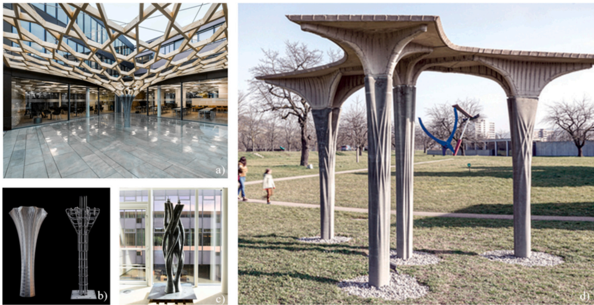
Fig. 22. a) Future Tree, Esslingen, Switzerland [81], b) Formwork for Future Tree [68], c) Post-tensioned columns with Eggshell [68], d) Vitra Pavillion [82].
