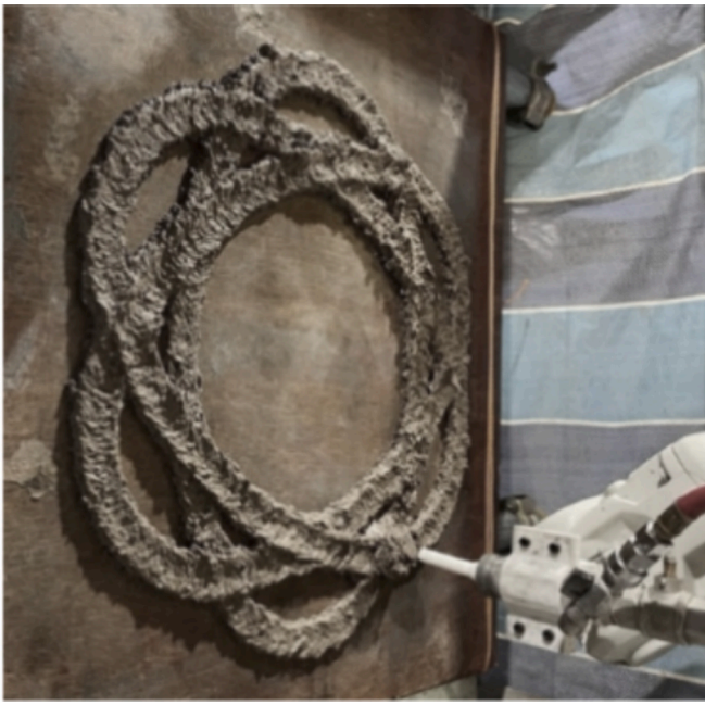
Fig. 8. Spray-based 3D Concrete Printing (S-3DCP, NTU Singapore, 2024) [31,32].
