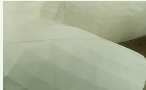
Figure 4.127: Filled seams after complete sanding.
