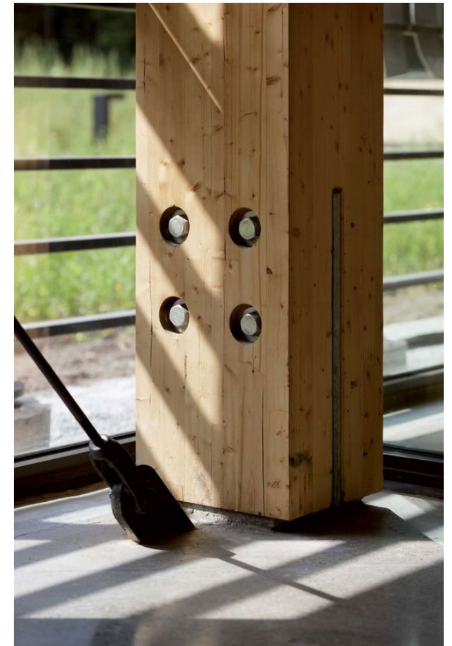
Connected with the concrete slab
