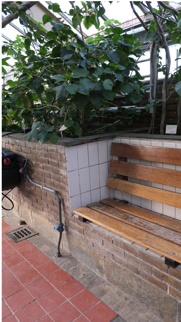
Brick works of plants bed
