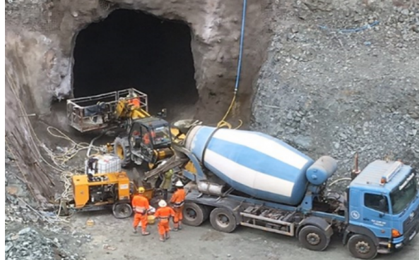
Figure 2.11: The initial work when the adit was first being opened.
