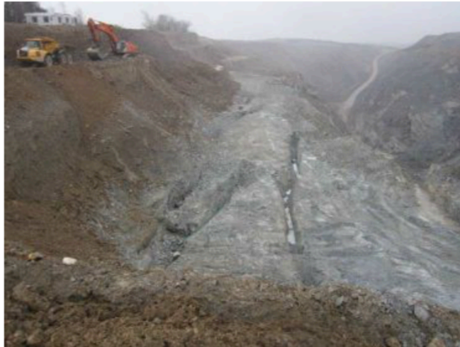
Figure 2.2: Kearney Pit post vein extraction (looking south, Volvo A40 for scale) (Phelps et al., 2014).
