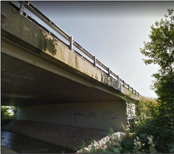
Figure 3. The Uerke Bridge (in a Google Street View).
