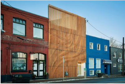
Junction 9 - MODA wooden half-open facade
