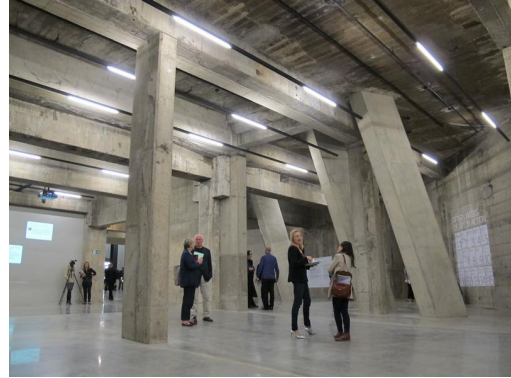
12 The Tanks at the Tate - Herzog and de Meuron - excavated basement - exposed concrete
