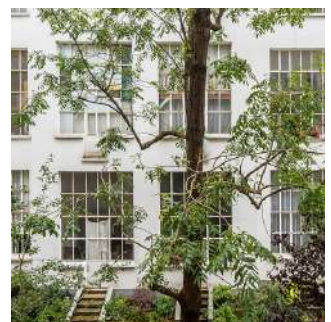
The atelier facade
