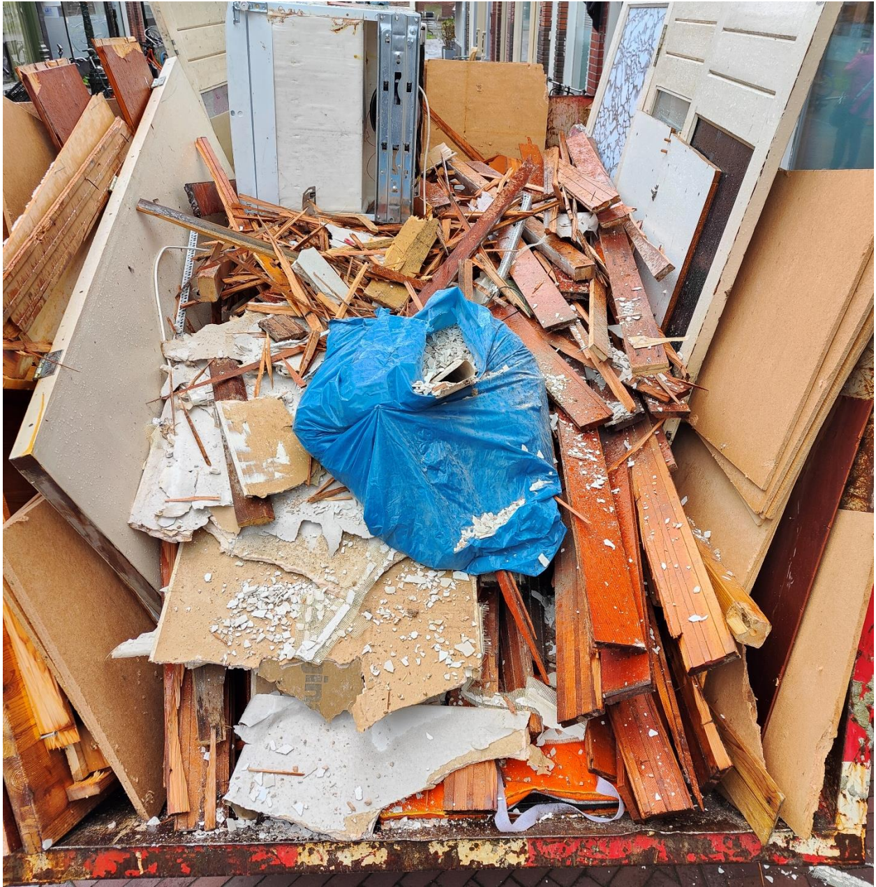
Figure A.2.7: 10 m 3 skip: wood, doors, refrigerator.
