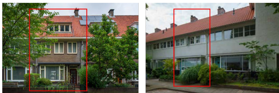
Figure 4. A typical terraced house constructed prior to 1945. The red box illustrates the dwelling’s intermediate (in-between) position within the adjoining row houses [67].
