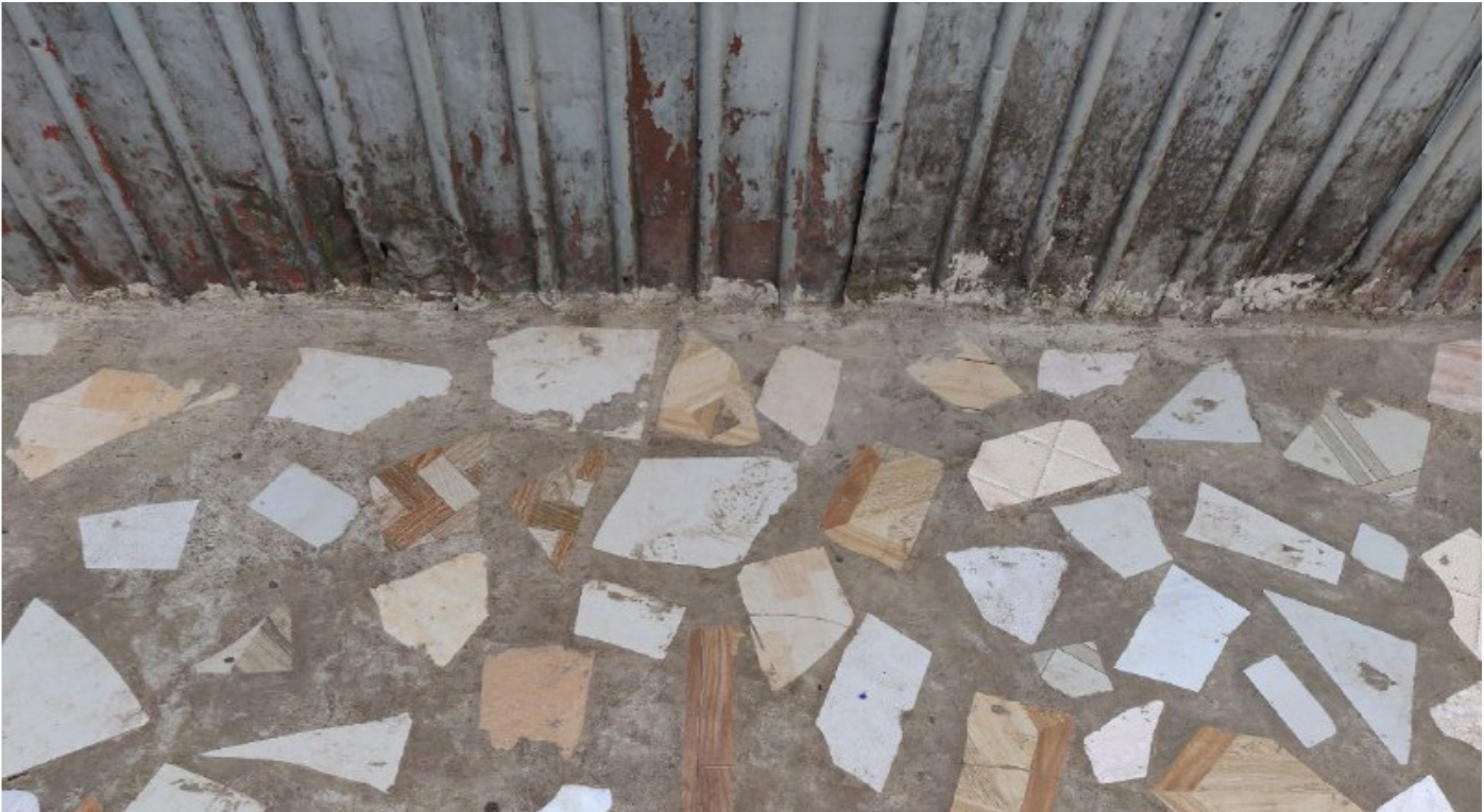
Broken tiles used in concrete for pavement in Kechene
