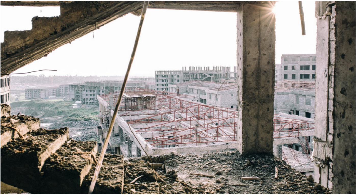
Concrete usage in the new condominium complex, Addis Ababa
