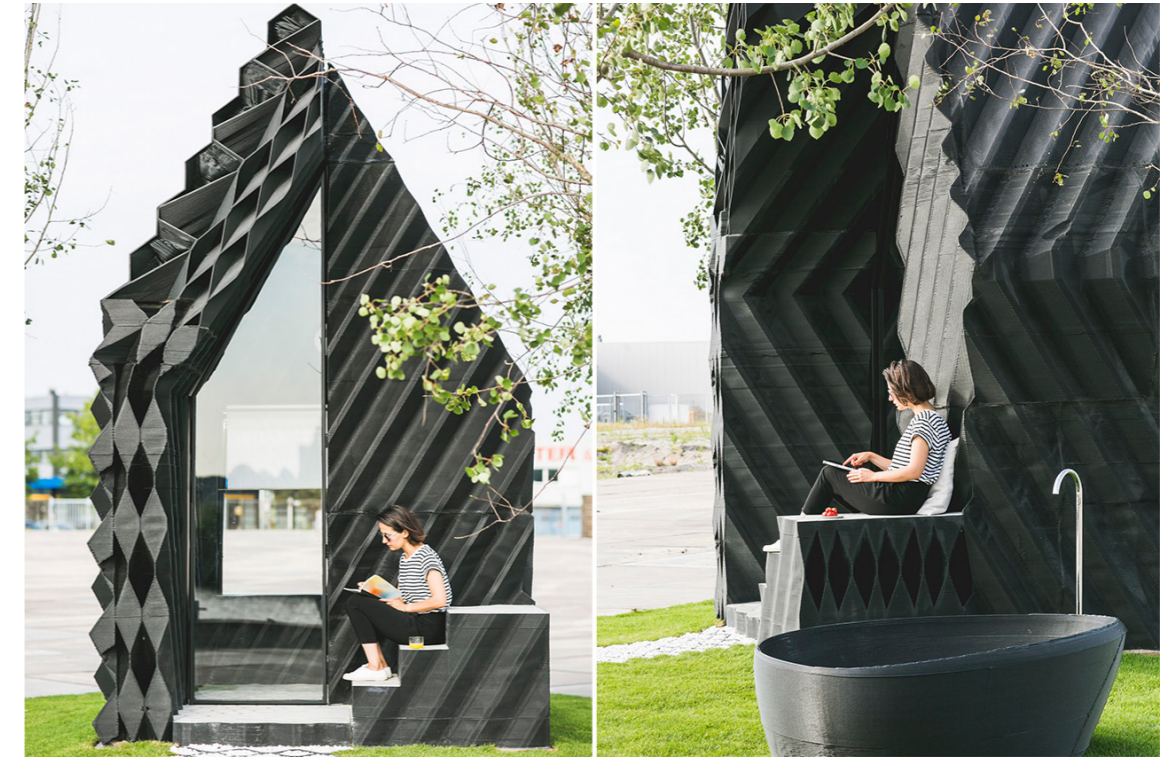
Figure 6. A fully 3D printed house in Amsterdam, designed by DUS Architects (van Duivenbode & van den Hoek, 2015)
