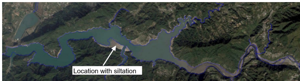
Fig. 4. Google Earth image of the Shihmen Reservoir at a moment with low water level in 2015. A location with siltation is indicated.
