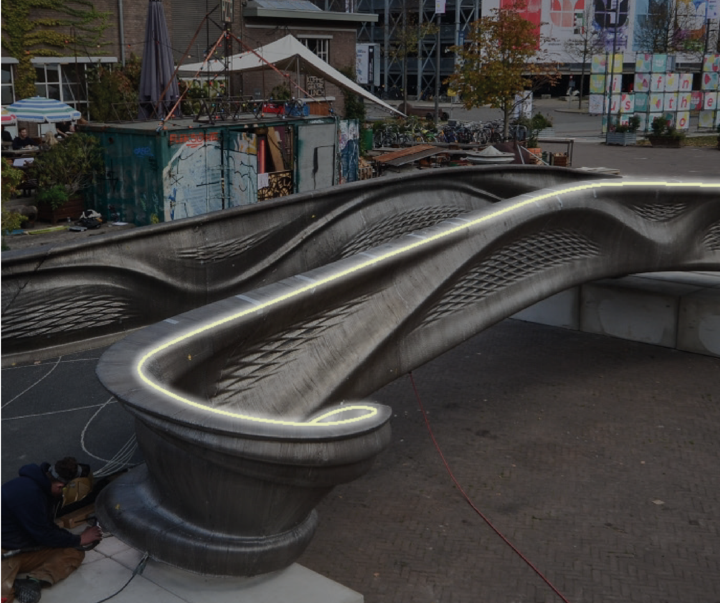
Figure I.2: MX3D bridge at the DDW 2018 showing the placement of the LED strip on side of the bridge.
