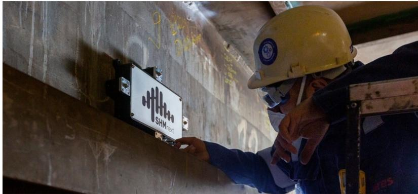
**Figure 1.14:** The UniQ of SHM Next applied to a bridge [12].
