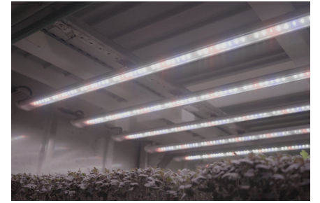
Picture 67: Lighting bars in the Urban Crop robotic solution at PLNT Antwerp
