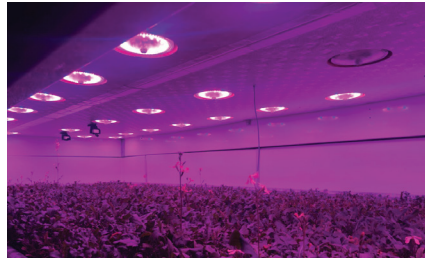
Picture 66: CEM with Pixel lights. The air is being exhausted around the LEDs
