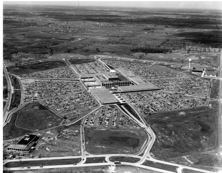
3.4 | Aerial view of Northland shopping centre
