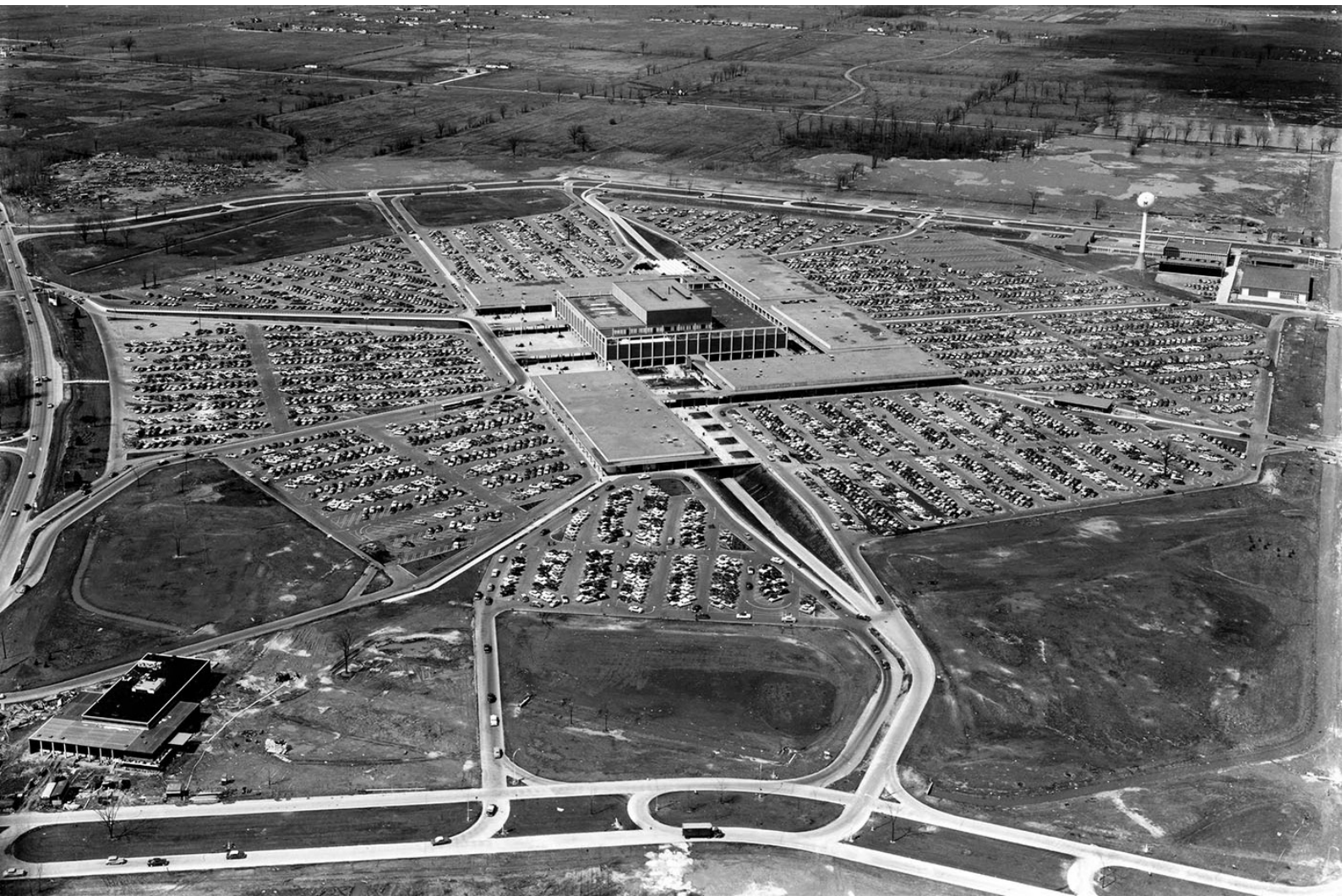
5.14 | Aerial view of Northland shopping centre
