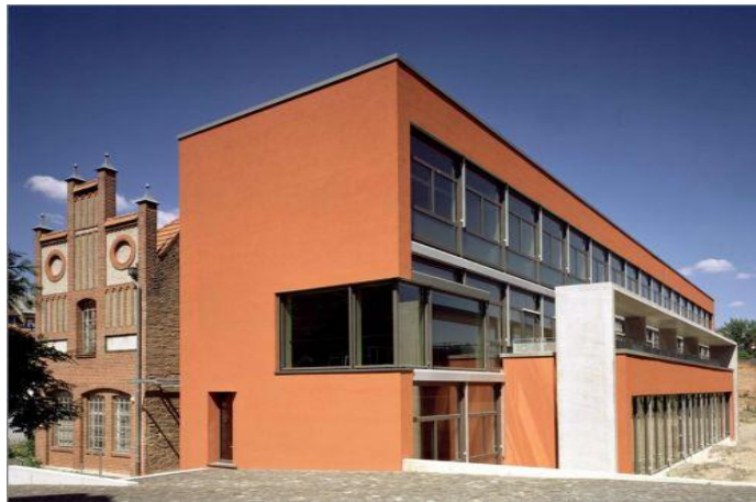
Figure 1. Test Case Building, Kassel Germany.
