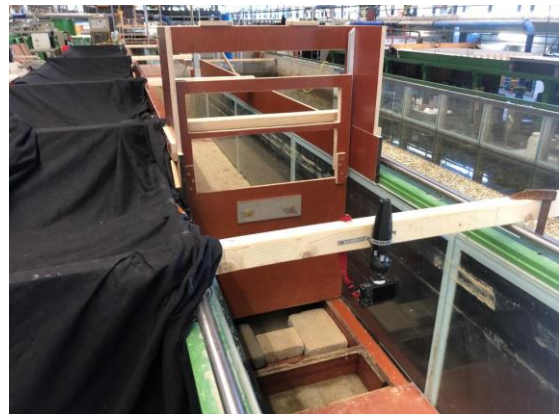
Falling gate and vertical lock construction.
