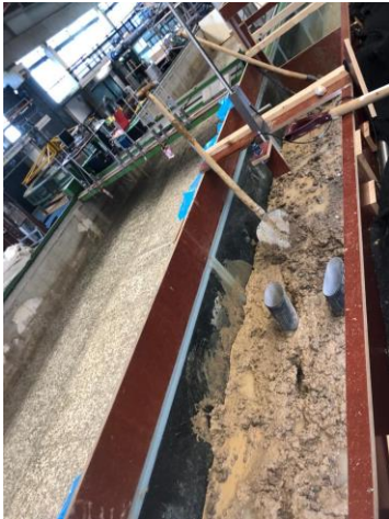
Preparation of the river clay package and installation of MIC 3.
