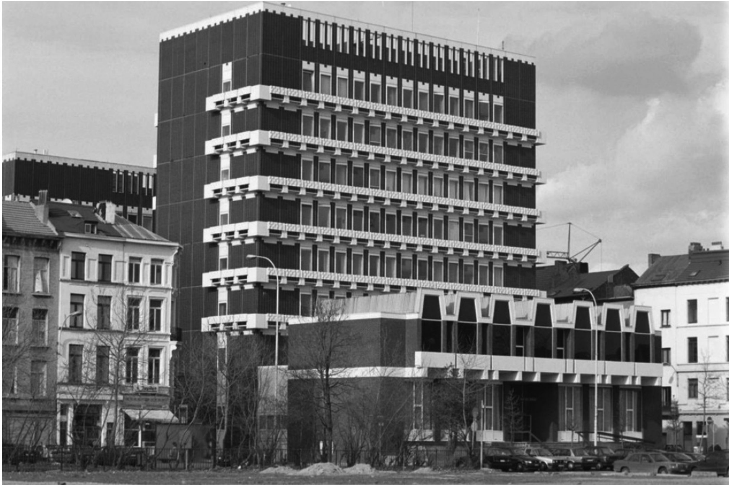
On the proposed site the old court house “Hof van Beroep” is located (VUM, 2014).
