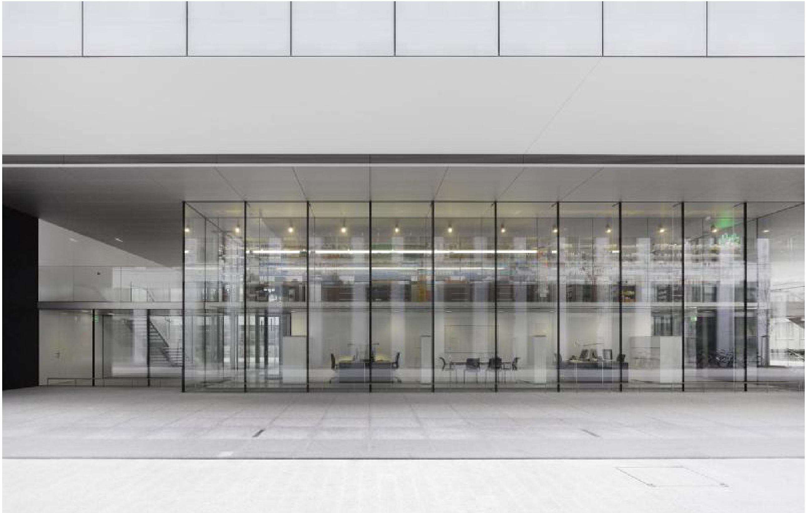
Open ground floor level of the Fabrikstrasse 10 in Basel by Yoshio Taniguchi (Johannes Marburg, n.d.)
