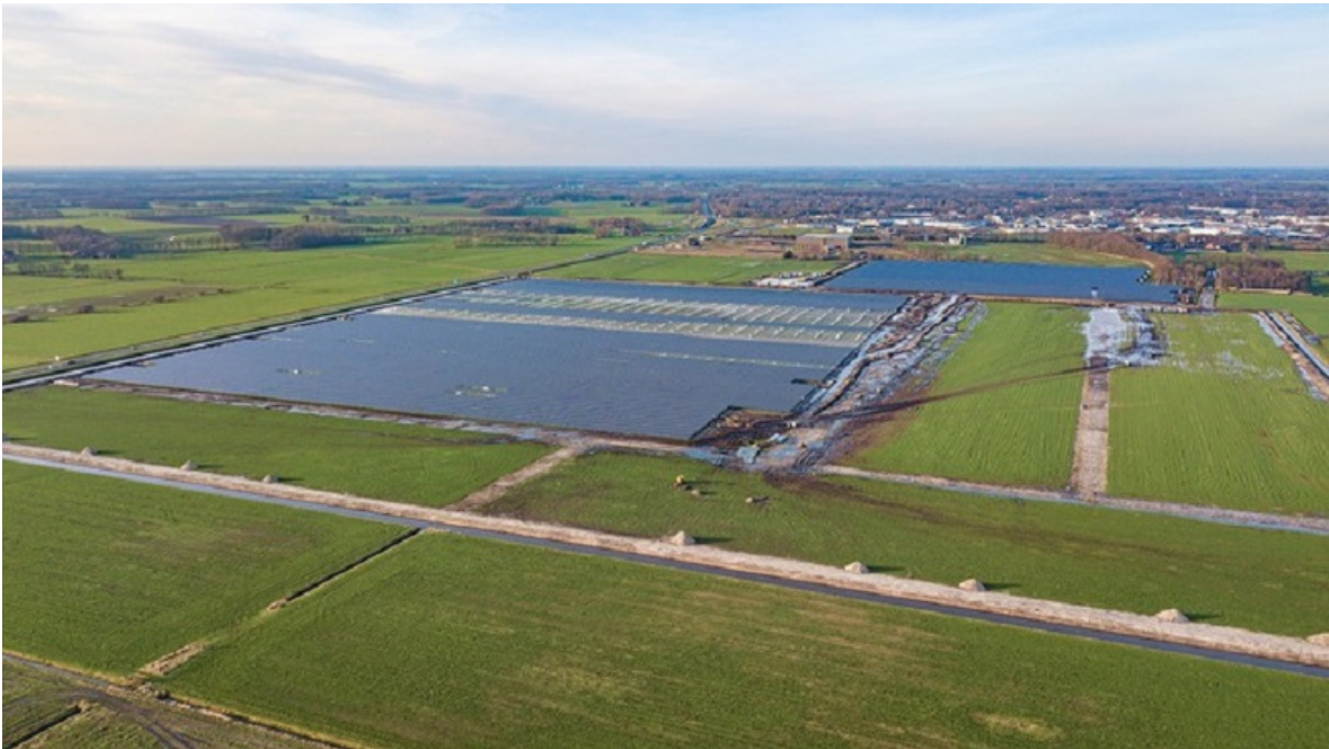
Figure 4.1: PV park Oosterwolde under construction.
