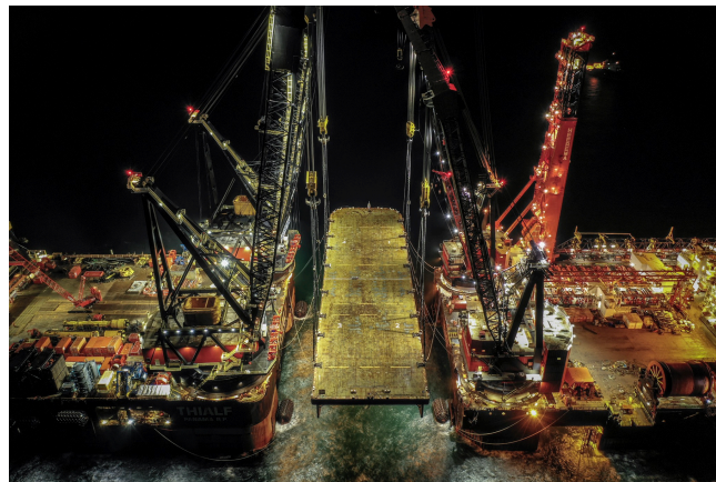
(b) SSCV Thialf & Balder performing the first QUAD Lift
