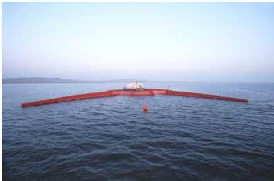
Figure 1.6: Overtopping Device Wave Dragon.
