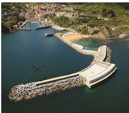
Figure 1.2: Integrated OWC power plant of Mutriku.
