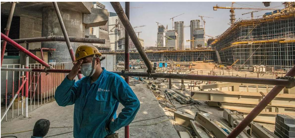
Fig. 19 Workers at the Iconic Tower skyscraper in 2021.
