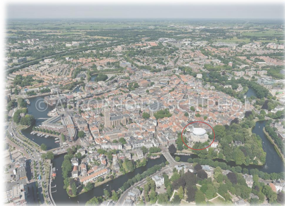
Figure 30: Air photo shows the relationship between the Fundatie and the idyllic city centre. Resource: www.aerophotostock.com
