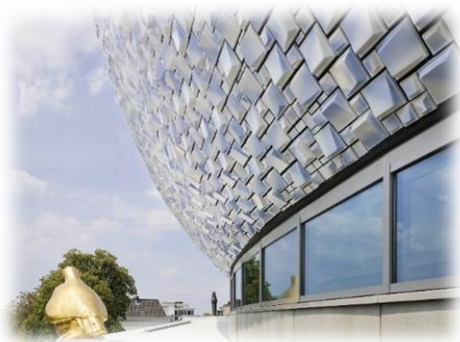
Figure 22: the counter between the existing building under and the upper new volume. Resource: www.biermanhenket.nl
