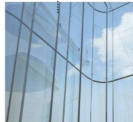
Insulated stick built glassfin curtainwall
