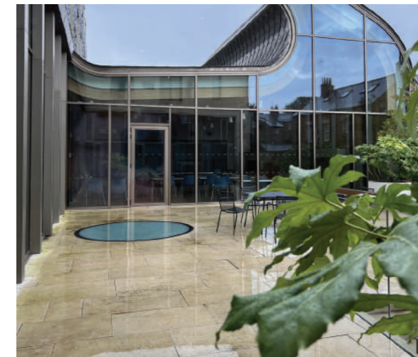
Back Courtyard of the Exeter College serves as reimagined quad introducing more visual connection between inside and outside, daylight and greenery.
