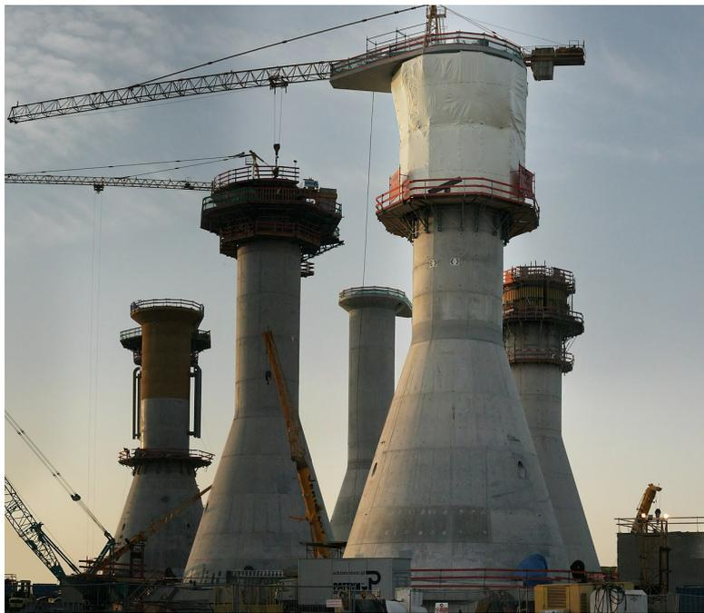
**Figure 1.7:** Gravity-based foundation under construction at Thornton bank offshore wind farm [7].
