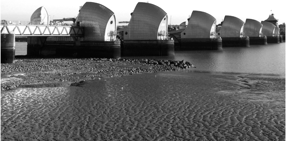
Figure 20 The Thames Barrier (photo by Author)
