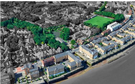
Figure 102 Large residential blocks with low quality riverfront access. Courtyards are used for surface parking
