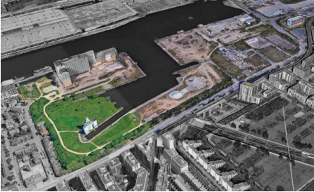
Figure 91 Large derelict industrial areas adjacent to Thames Barrier Park, currently set for redevelopment
