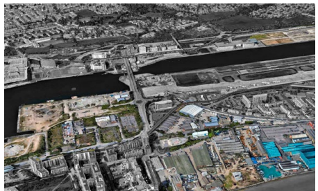
Figure 96 Derelict industrial facilities and London City airport
