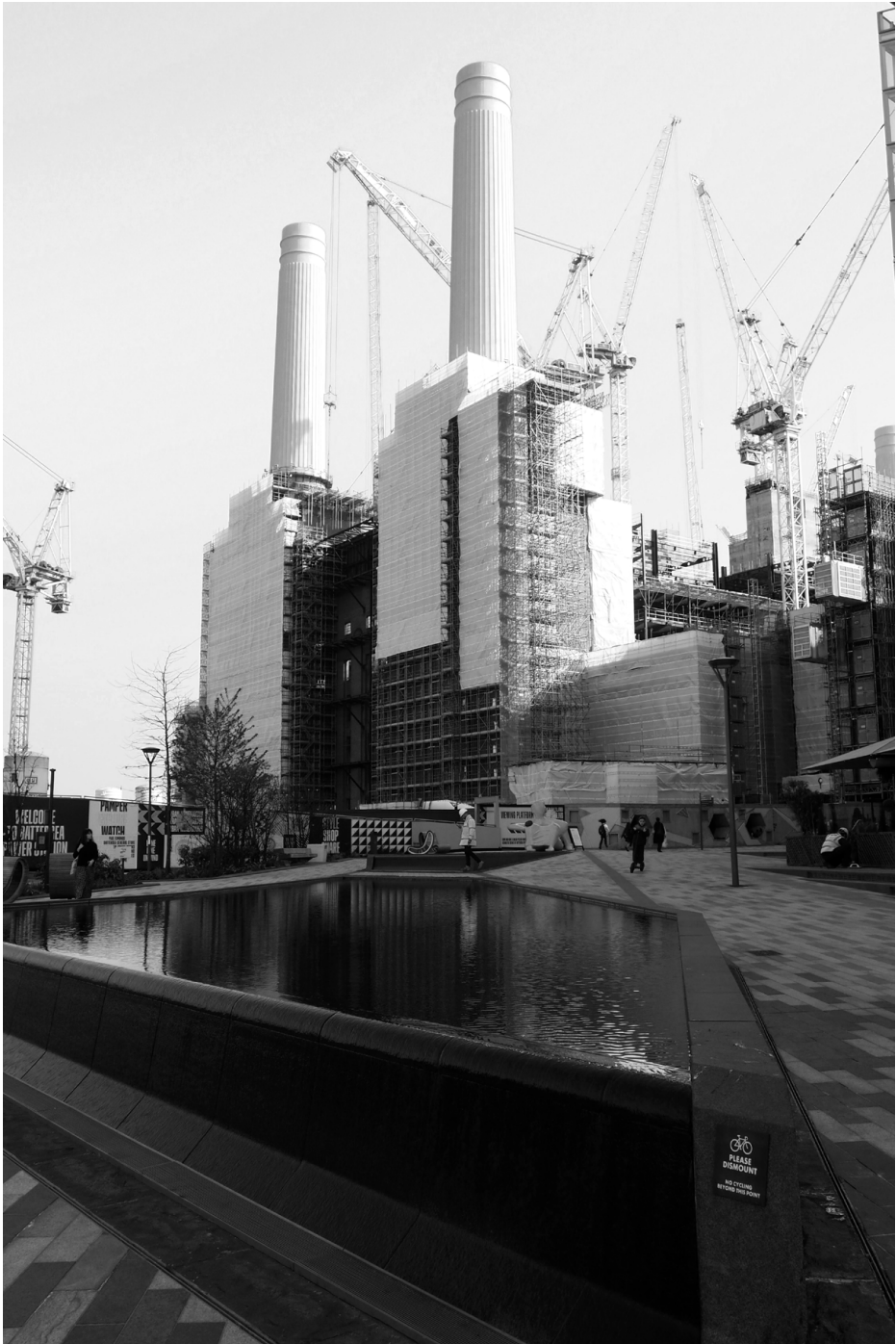
Battersea Power Station, Photo by Author
