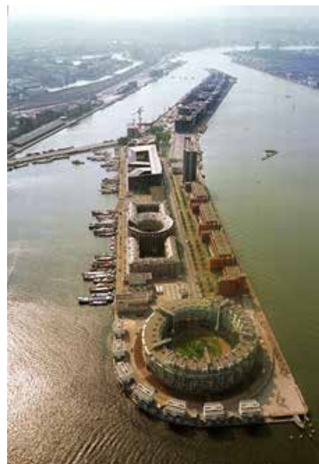
KNSM-Island finished (Amsterdam Archief, viewed at april 4 2022)
