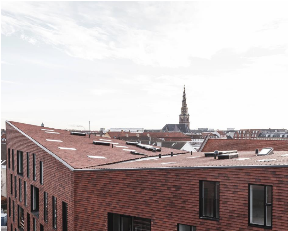
Fig. 60. The new roof with the same height as the neighbouring buildings (Cobe, retrieved April 22, 2022).
