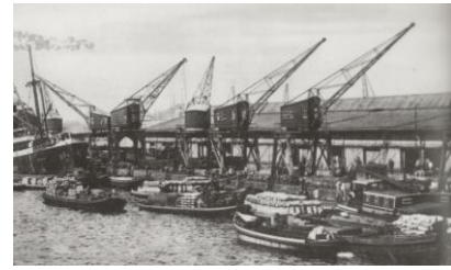
Figure 6. Cranes on the Leventkade, approx. 1920 (Stadsarchief Amsterdam, retrieved April 3, 2022).
