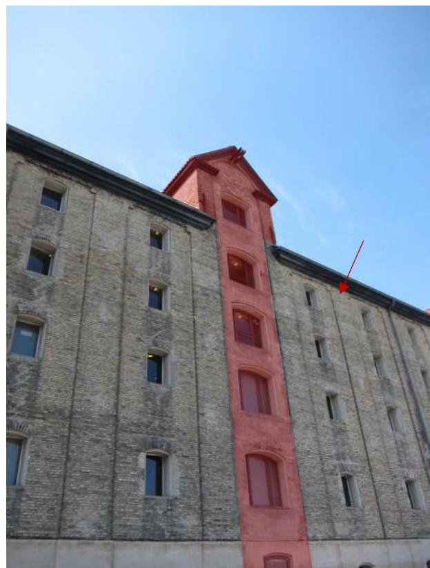
Figure 15. The large Warehouse, (now called North Atlantic House) from 1766 in the distinctive style Lisen (from Latin licium , French lisse , "thread", "band") inspired by architect Nicolai Eigtved (1701-1754) is called the building art of a flat but slightly prominent pilasters use of which only has decorative function. The middle part was used for lifted goods into the building (Kulturministeriet, Slots- og Kulturstyrelsen, 2016).
