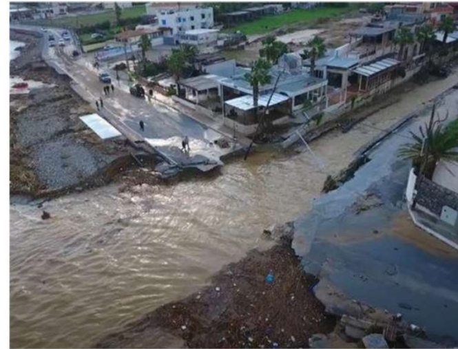
Flooding events in Crete, 2020, Municipality of Hersonissos, Gouves
