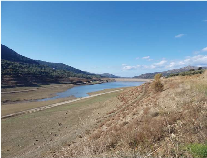
Extremely low water level - Aposelemis dam, December 2023
