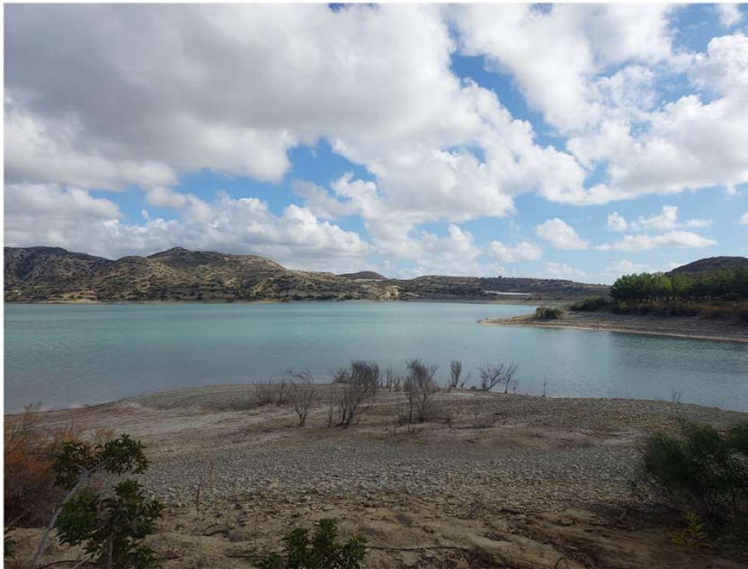
Bramiana dam extremely low water level, December 2023
