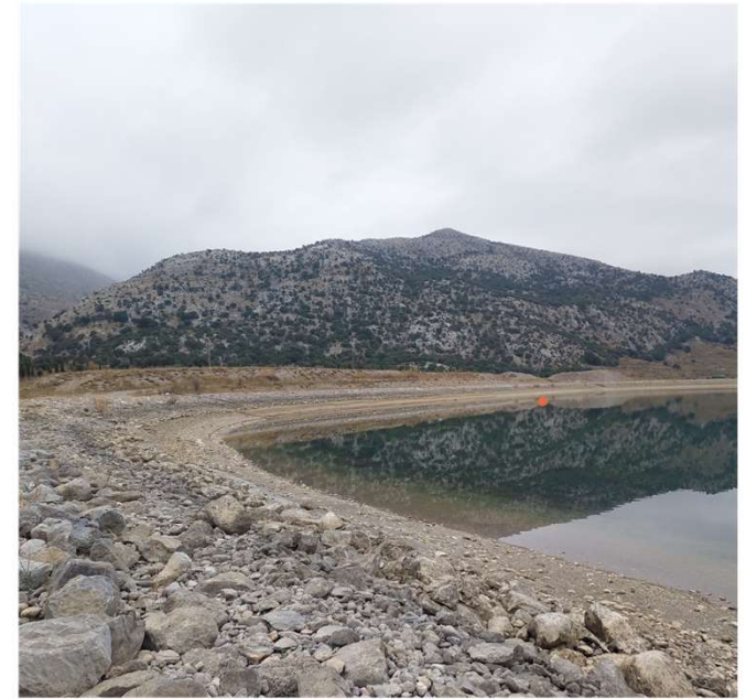
Low water levels of water reservoir at Lasithi, created to prevent from flooding and collect the water for agricultural water supply, 2023
