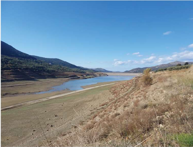
Extremely low water level - Aposelemis dam, December 2023
