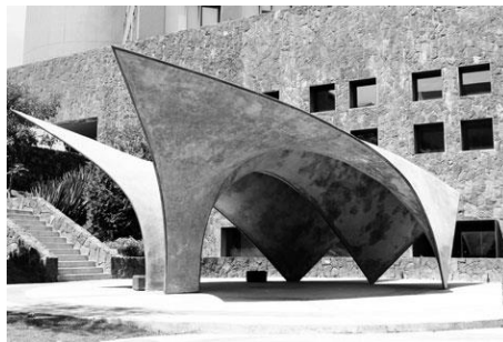
Figure 2.6 : Cantilevering concrete shell canopy, Mexico City, Mexico, 2011 (photo credit: (Adriaenssens et al., 2014))
