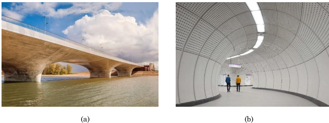
Figure 2.9: Examples of structures realised using the subtracted formwork method: (a) The Extended Waalbridge by ZJA, Nijmegen, The Netherlands, 2015; (b) The Elizabeth Line by Grimshaw, London, United Kingdom, 2019; (photo credit: (a) Raymond van der Hoogt; (b) Grimshaw).
