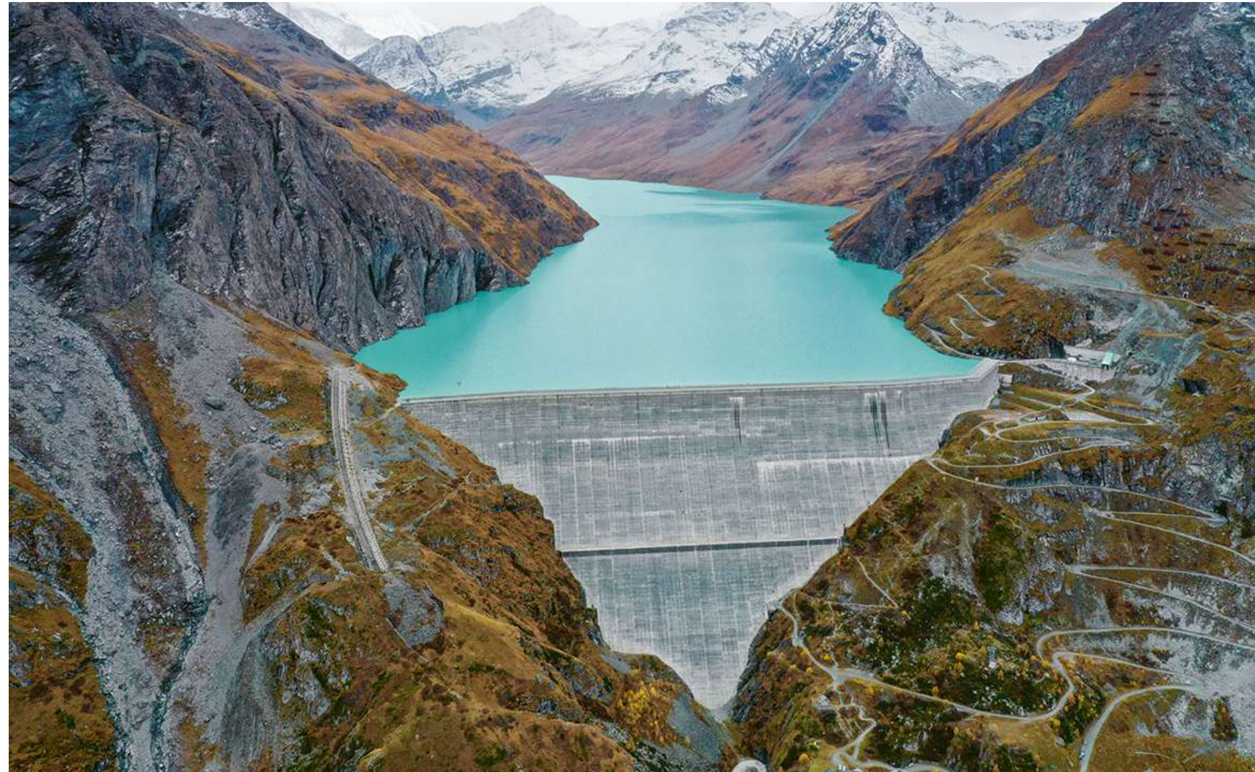
Dammed river in Switzerland (Jérémy Toma)
