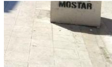
Limestone and concrete paving in Mostar
