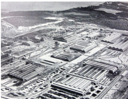
FIG. 1.8 Aerial view of the new city center of Ciudad Guayana, in the sector of Alta Vista, during its construction in the 1960s. Source: Rodwin, 1969.
