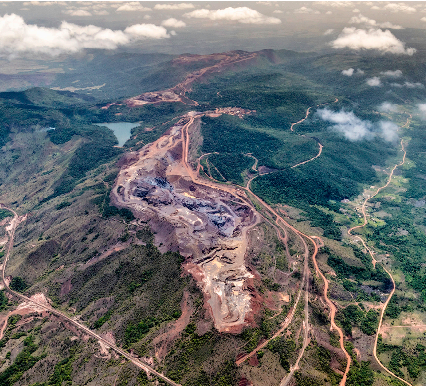
FIG. 1.1 The discovery of iron ore deposits in the Venezuelan Guayana prompted the construction of several company towns by American mining corporations during the 1940s. Some years later, the democratic government of Rómulo Betancourt decided to plan the industrial new town of Ciudad Guayana to diversify the national economy, based on the extraction and processing of natural resources. In this image, the iron ore deposits of San Isidro, near the new town of Ciudad Piar. Retrieved from https://clarknow.clarku.edu
