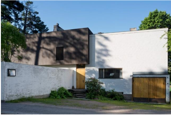
Figure 14: Entrance of the Aalto House (1936), Alvar and Aino Aalto.
