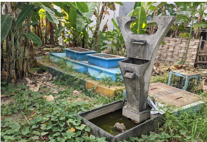
Figure 3. Greywater treatment system from the community dining hall in Kelurahan Jambangan, Surabaya.
