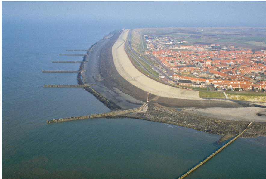
Figure 10.28: Sea dike, Westkapelle, the Netherlands, in June 1993. From Rijkswaterstaat ('Credits' on page 575).
