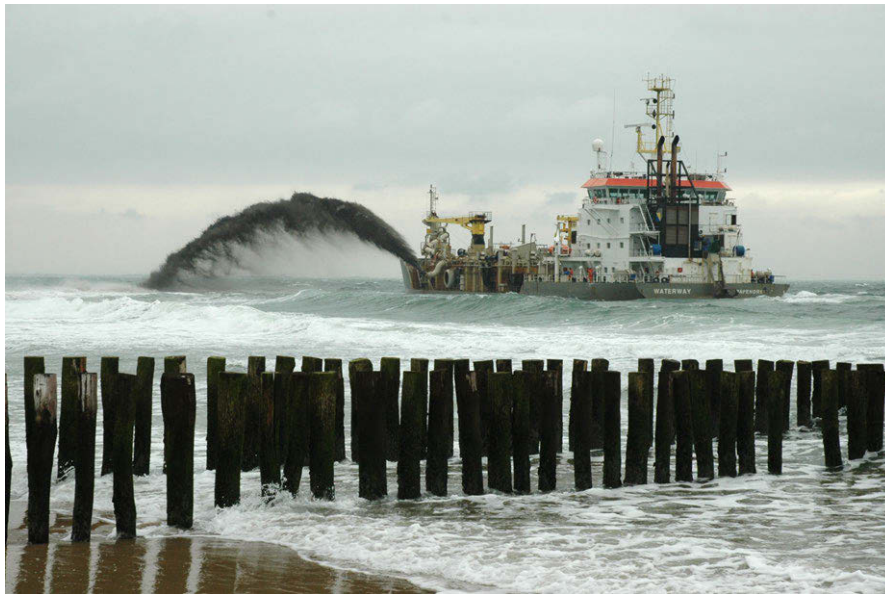
Figure 10.33: Shoreface nourishment at the Dutch coast through rainbowing in September 2005. From Rijkswaterstaat ( ‘Credits’ on page 575 ).
