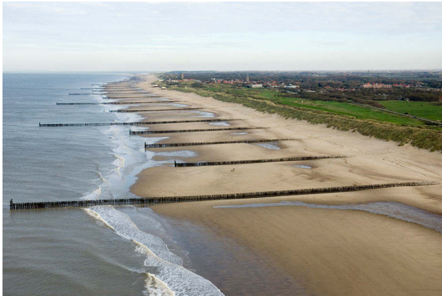
Figure 10.13: Groynes on the Dutch southwestern delta coast, near Domburg, in November 2005. Photo from Rijkswaterstaat ( Credits on page 575).
