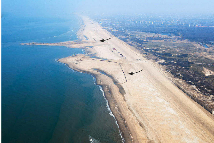
Figure 10.32: Beach suppletion during construction of the Sand Engine using pipelines (indicated by the black arrows) that cross the breaker zone in March 2011. From Rijkswaterstaat ( ‘Credits’ on page 575 ).
