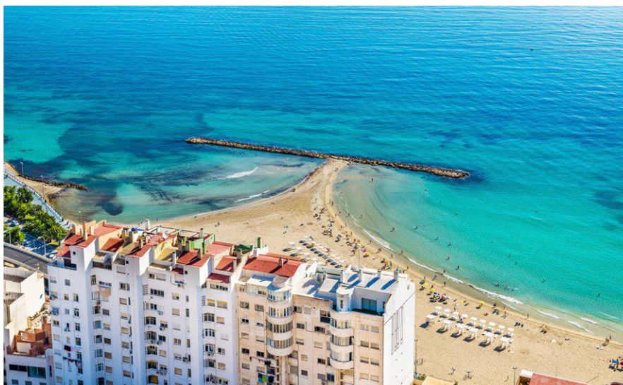
Figure 8.21: Tombolo formed behind a detached breakwater in Alicante, Spain. Photo by Leonid Andronov ('Credits' on page 575).
