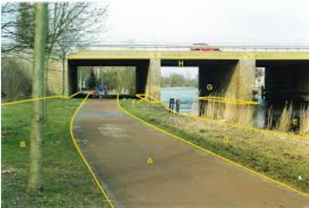
Figure 1: Relative height information as available in the BGT. The bridge (H) is at relative height level '1'. The bridge-parts F and G as well as the road, verge and water are at relative height level '0'. The latter form a planar partition (IMGeo, 2020)
