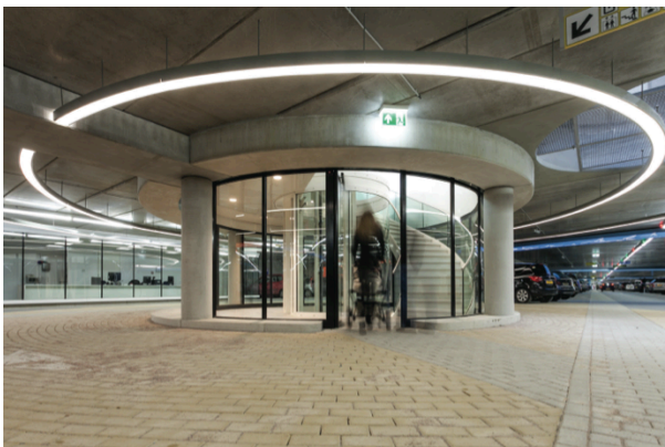
Figure 77 Pavement floor in the parking garage to maintain access to the drainage system underneath
